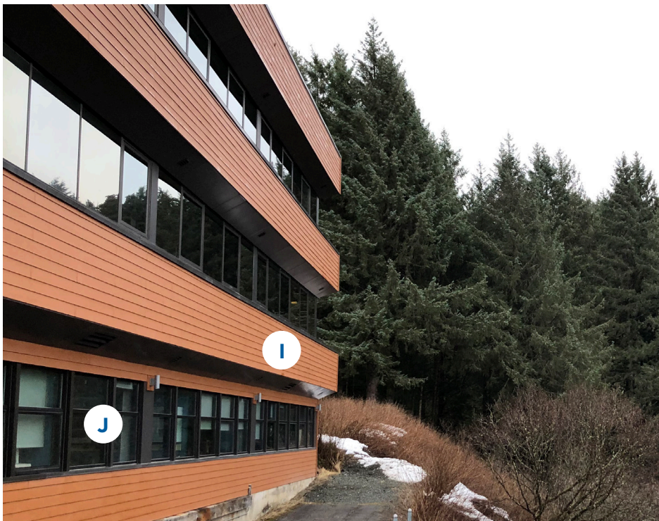
Anderson Building, side facing Auke Bay Photograph by UAS
